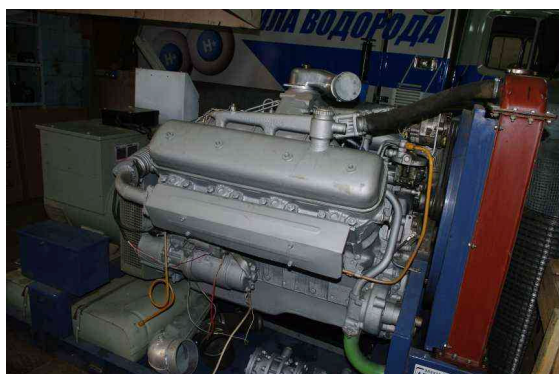
Figure 8: NAMI power plant
